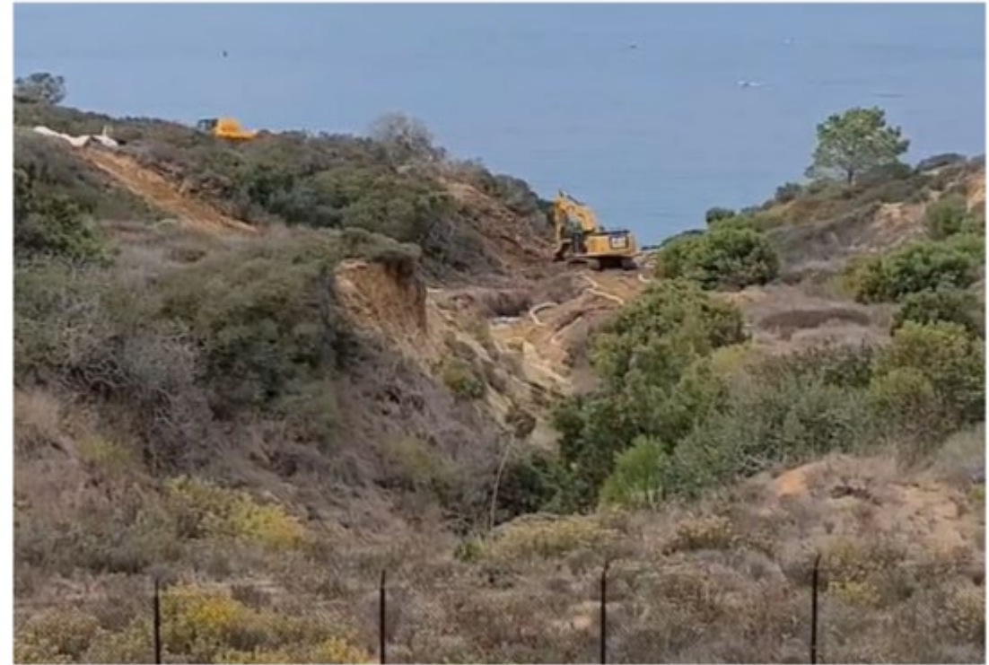
View of site from Cabrillo Memorial Road (facing west) (Jacobs n.d.)
